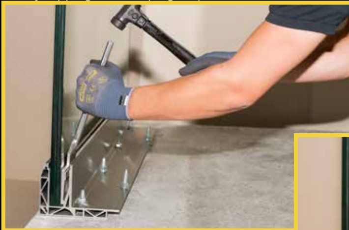
Gently tapping the clamping strip
